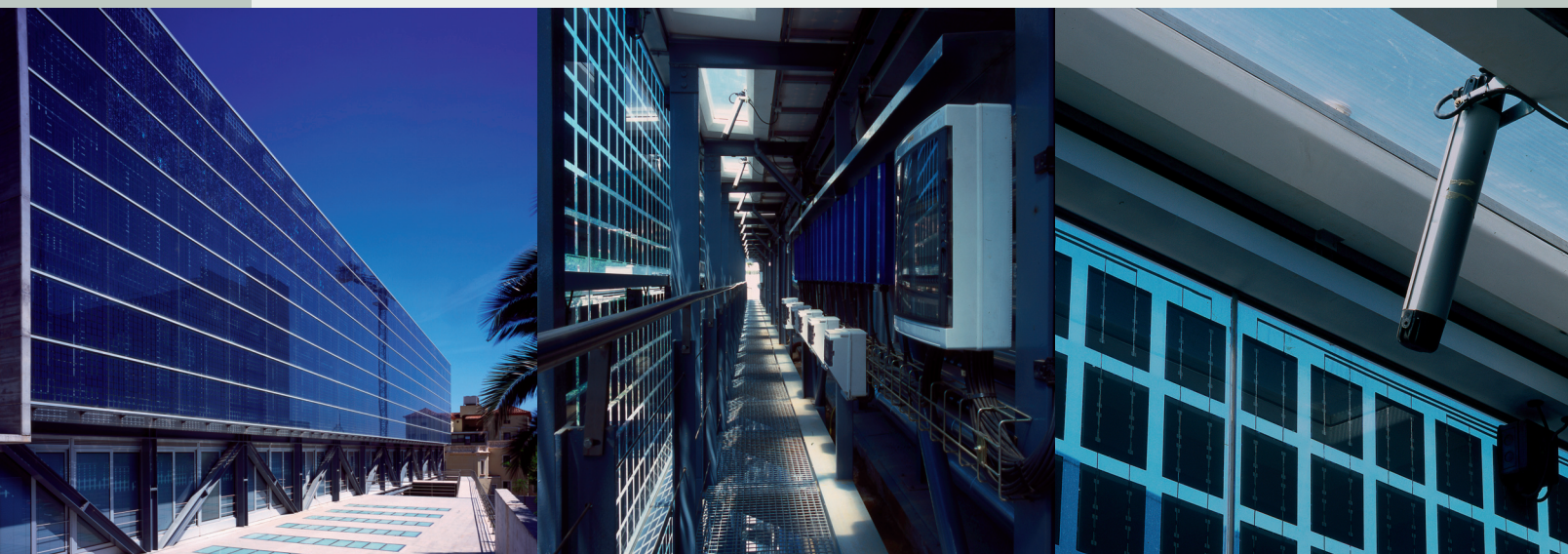
Curtain wall with photovoltaic panels - La Salle - Barcelona, Spain (Architect : Robert y Esteve Terradas Muntañola)
